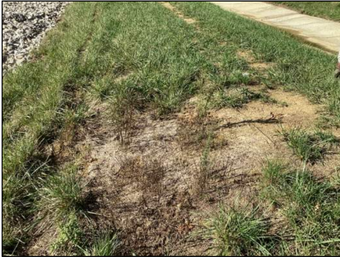
Photo 10, Point 10 Southwest Sediment Basin – Bare spot with mulch on slope.
