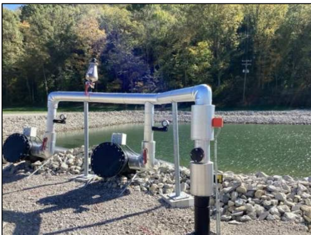
Photo 21, Point 21 Southwest Leachate Pond – Pump piping.
