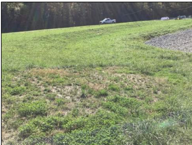
Photo 17, Point 17 Southwest Sediment Basin – Bare spot.
