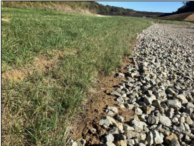
Photo 8, Point 8 Southwest Sediment Basin – Sloughing on inside slope.
