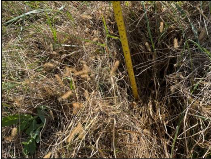
Photo 58, Point 58 Phase 1 – Depression (16 in. deep max.) on northwest slope temporary cover.
