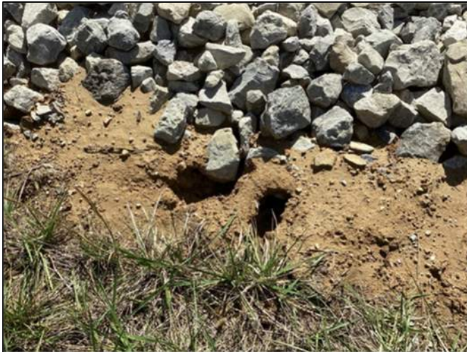
Photo 38, Point 38 Northeast Sedimentation Basin – Small holes on inner slope.
