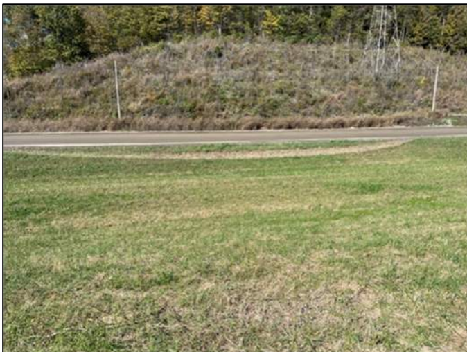
Photo 60, Point 60 Phase 1– Dead vegetation from large tire track on north slope temporary cover.
