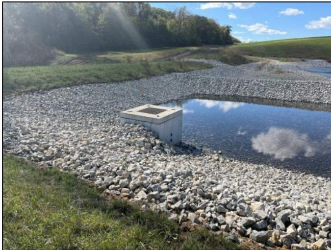
Photo 44, Point 44 Northeast Sedimentation Basin – Riser/inlet structure.
