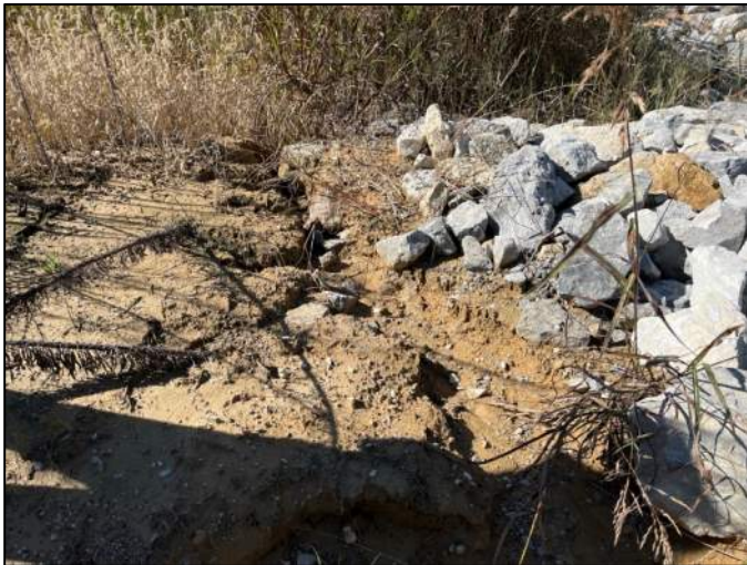
Photo 32, Point 32 Erosion channel (18 in. deep max.) outside of riprap-lined area.
