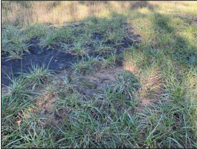
Photo 28, Point 28 Bare spot with exposed TRM near stormwater channel.
