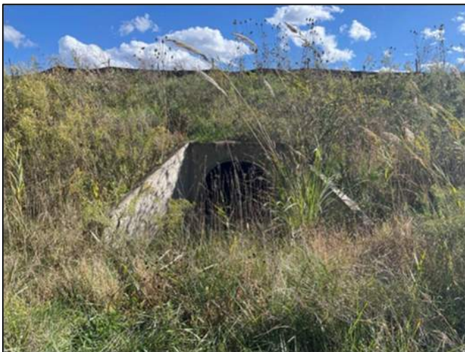
Photo 75, Point 75 Vegetation around culvert to diversion ditch.
