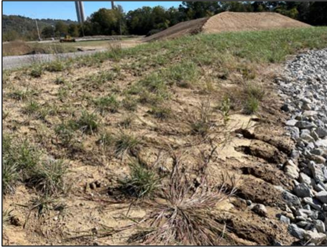
Photo 37, Point 37 Northeast Sedimentation Basin – Bare spot and erosion rill on inner slope.
