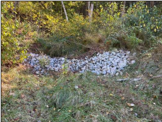
Photo 29, Point 29 Check dam of stormwater channel is washed out.
