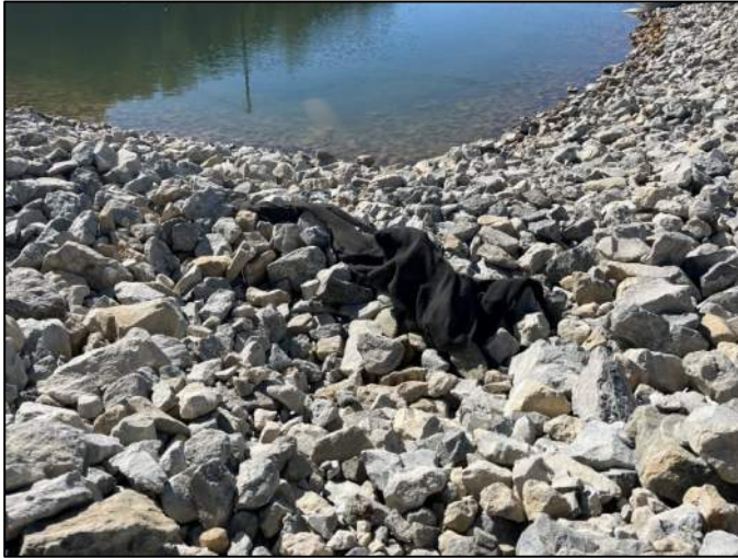
Photo 22, Point 22 Southwest Leachate Pond – Geotextile fabric exposed in riprap protection on northwest corner.
