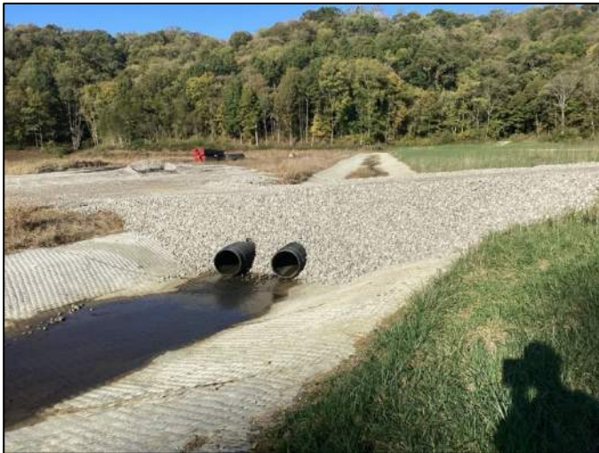
Photo 23, Point 23 Lined stormwater channel crossing outlet adjacent to Southwest Leachate Pond.
