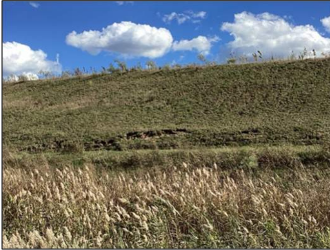
Photo 67, Point 67 Scarp on stockpile located north of Northeast Sedimentation Basin.
