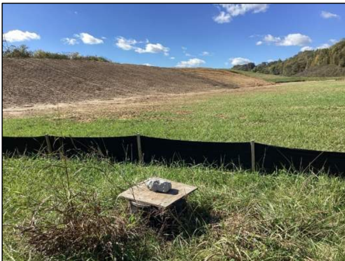
Photo 36, Point 36 An estimated 24-inch diameter standpipe located west of Northeast Leachate Pond and stockpile in the background.
