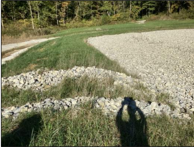
Photo 7, Point 7 Southwest Sediment Basin – Emergency spillway to lined stormwater channel.
