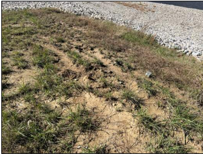
Photo 43, Point 43 Northeast Sedimentation Basin – Bare spot and erosion rill on slope.
