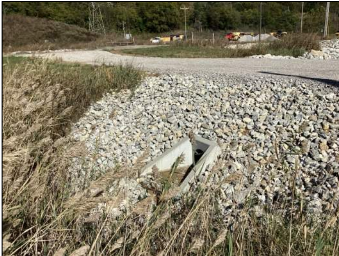
Photo 35, Point 35 Stormwater channel inlet headwall north of Northeast Leachate Pond.
