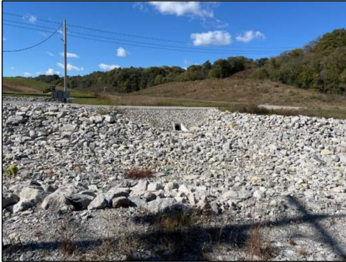
Photo 31, Point 31 Stormwater channel outlet into riprap-lined ditch east of Northeast Leachate Pond.
