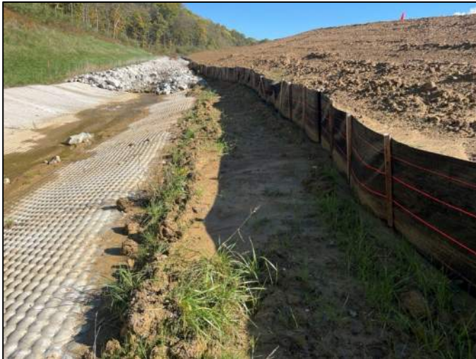
Photo 14, Point 14 Bare spot on slope and riprap in lined stormwater channel.
