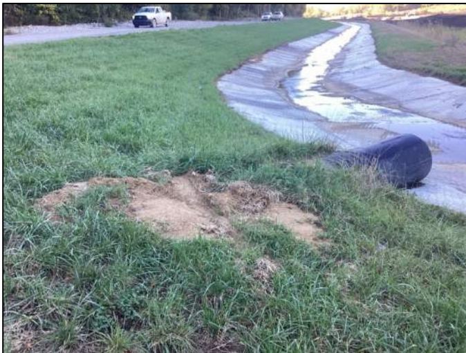
Photo 24, Point 24 Bare spot above pipe outlet to lined stormwater channel.
